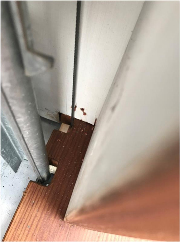
East shutter axle cable threading and track cover
