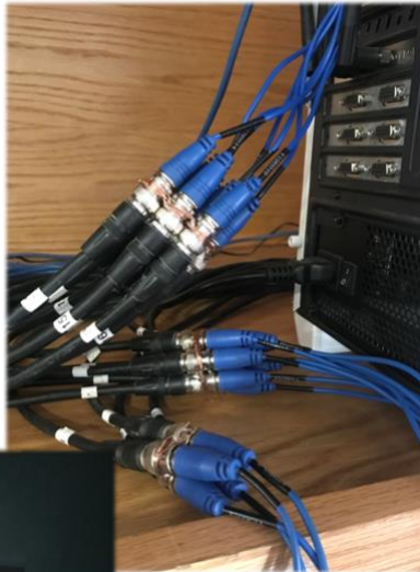
CAMS video grounds tied and chassis-bonded to reduce noise
