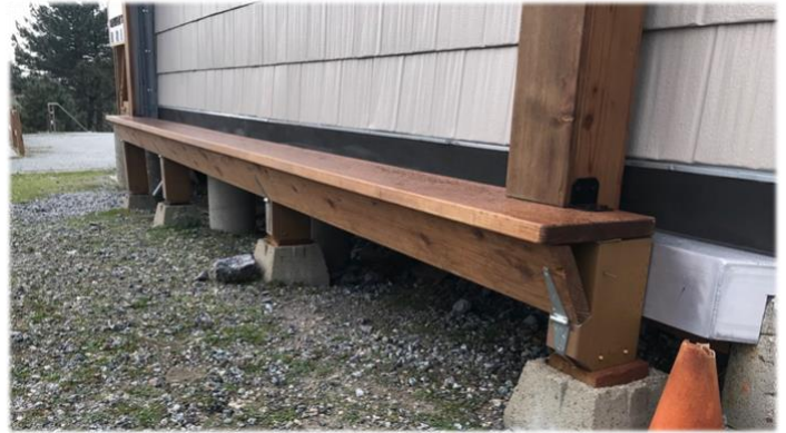
New bench and shutter axle cover/lower support
